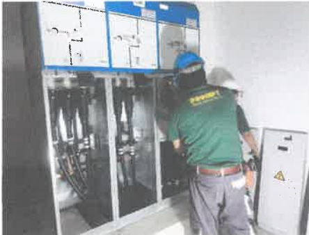
Medium Voltage Switch Gear Preventive maintenance
