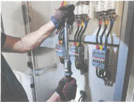
Capacitor Bank Preventive maintenance tighten the screw
