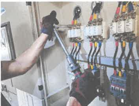
Capacitor Bank Preventive maintenance tighten the screw
